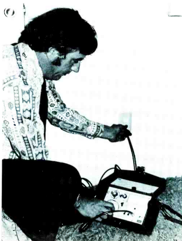
Fig. 17 Bob Polley, Sales Manager for National Comco, is pictured checking the video and audio carrier levels of each channel at one tap-off.
