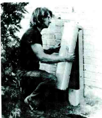
Fig. 14 Metal, weatherproof pedestals outside each building house and protect splitters and amplifiers.
